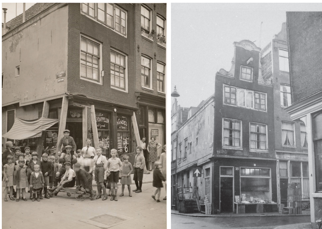
Figure 6. Example of modifications to a house (Bloemstraat 35). Original building with late 17th/early 18th century gable. To the left photo dating to 1930, with a lower facade timber frame probably dating the 19th century suffering from structural problems. To the right a photo from the 1950s, showing the replaced lower facade with a different window and door configuration (both images: Stadsarchief Amsterdam 4 ).
